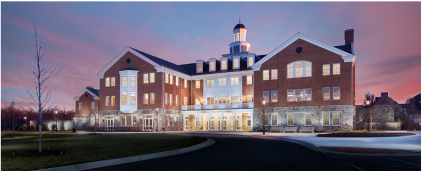
The Edward St. John Learning Center, located on the campus of McDonogh School in Owings Mills
